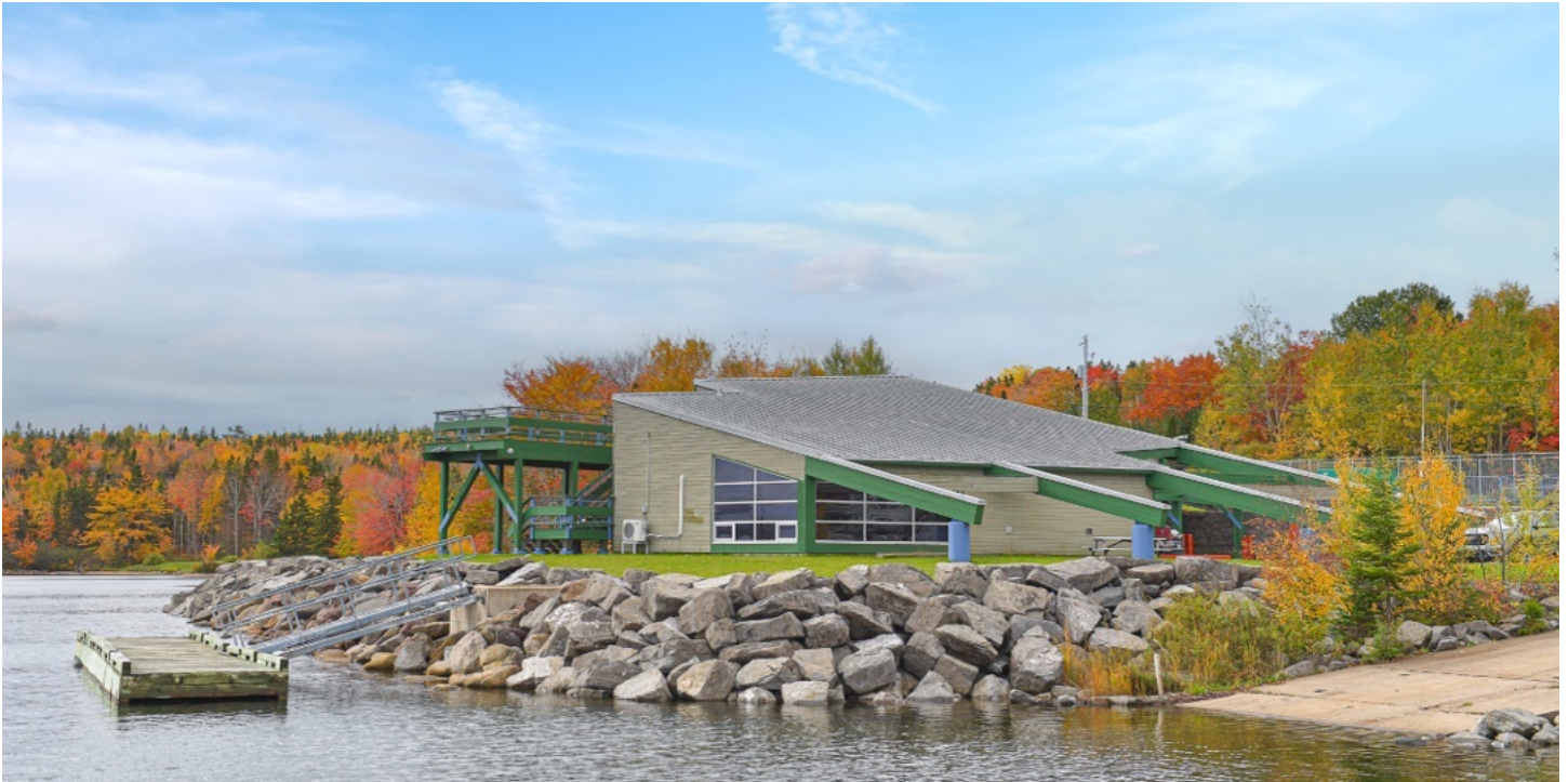
Current view of Wagmatcook Wharf
